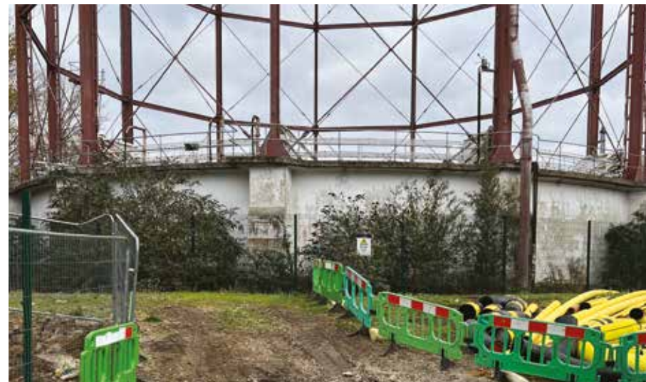
Existing gas holder structure
