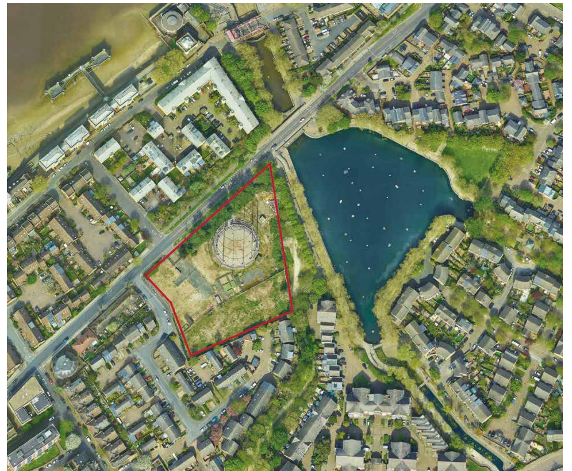
Aerial view of the site
