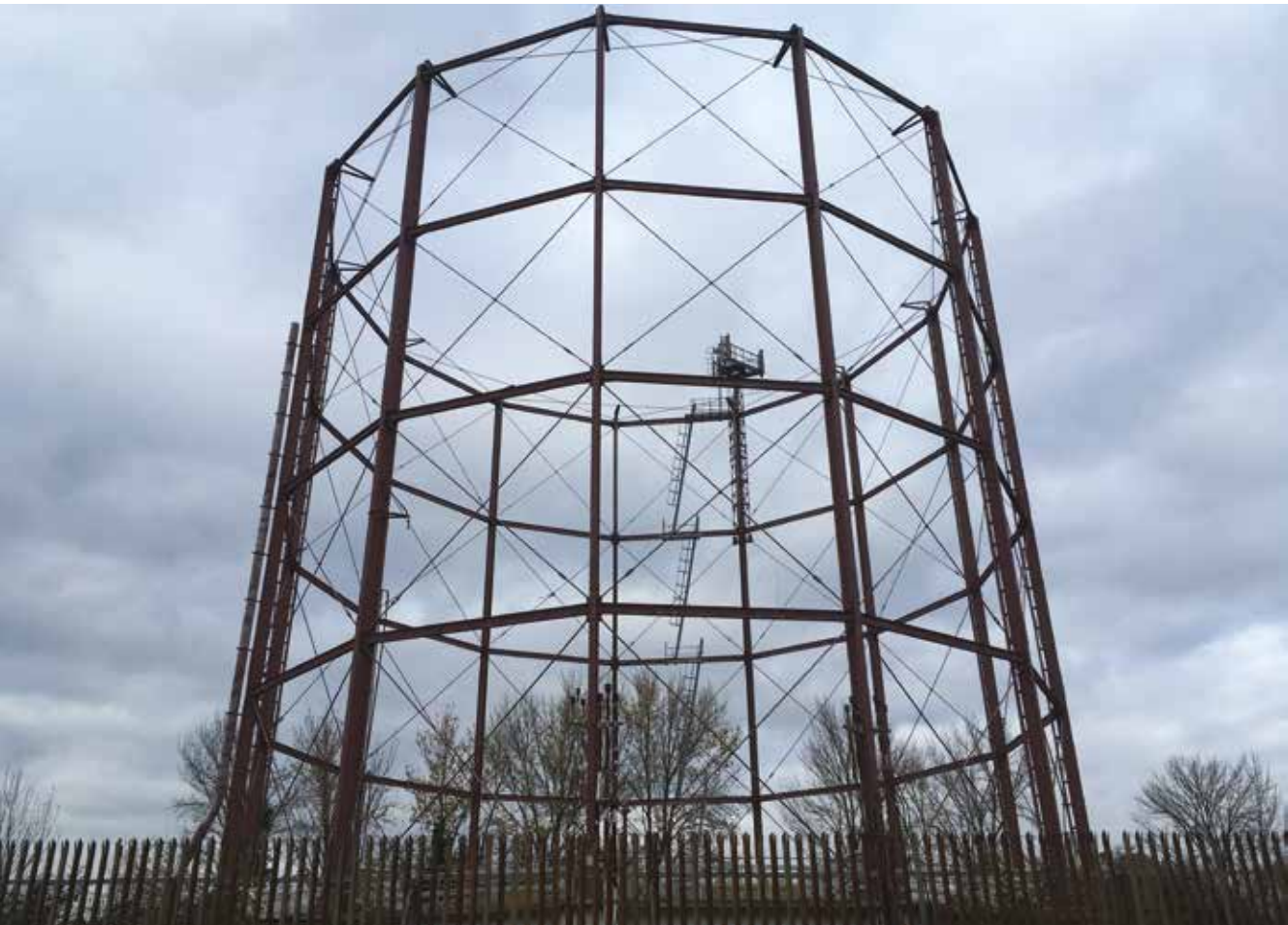
Existing gas holder structure on site
