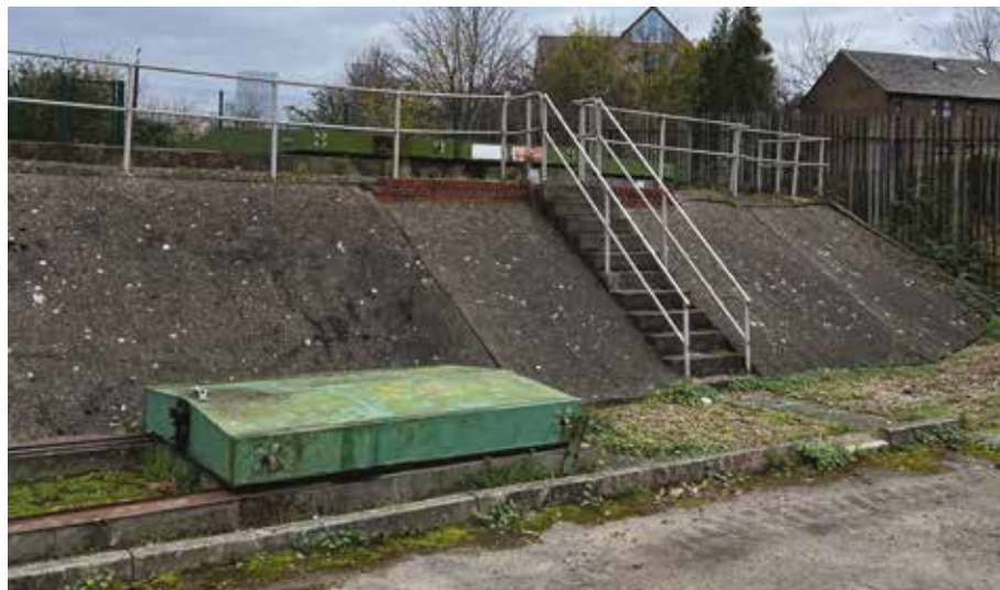
Existing gas infrastructure
