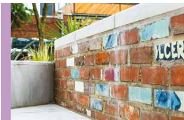
Seating wall from recycled block
