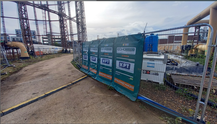
Acoustic barrier around generator to reduce noise output
