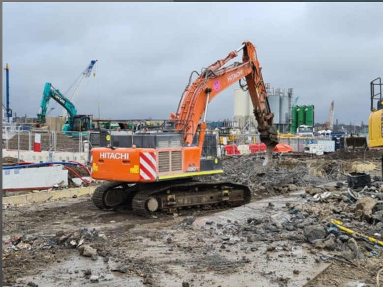
Use of plant with 'ripper tooth' attachment to pull at concrete slabs, which will then be processed using munching attachments to reduce noise and vibration
