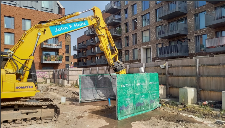
Acoustic barrier around generator to reduce noise output
