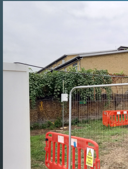
Real time environmental monitor in place on boundary to site, near to closest residential receptors.
