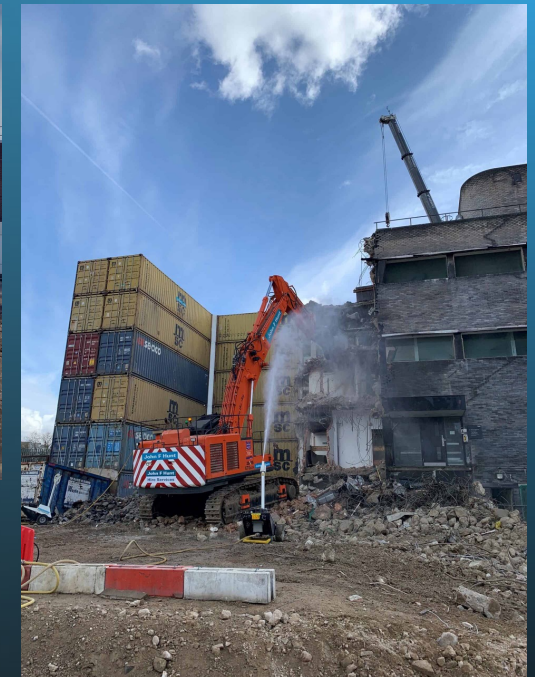
Dust suppression on high-risk dust generating works.
